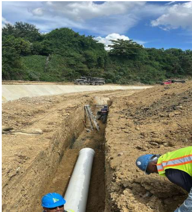
tuberia 16" pvc colectora
